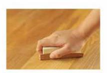
Sand the seasoned wooden surface using emery paper (180) along the grains. Repeat the sanding smoothly with finer grade of emery paper (220/320) and then wipe off the loose dust particles. Apply the coatings as follows:
